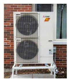
The Zuba Central system is the perfect solution for our cold Canadian climate. Performing best at low temperatures, it provides 80% of its rated heat at -25°C, meaning it operates superior to other central heat pumps. Thanks to this much heat being generated efficiently at low temperatures, the inefficient backup electric heaters will rarely be used, if at all. The Zuba Central also provides efficient cooling.
