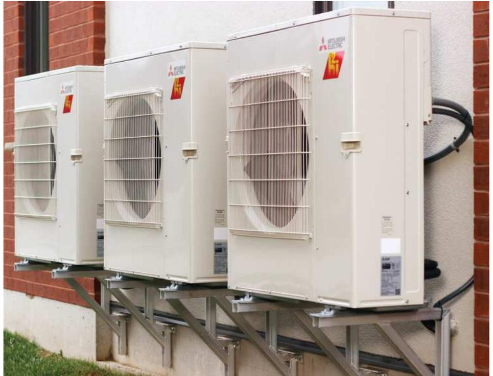
Part of the Zuba family of Mitsubishi Electric products, the centrally ducted cold climate air source heat pump system chosen features 100% output at  $-15^{\circ}\text{C}$ , which is substantially better than previous product in phase 1.
